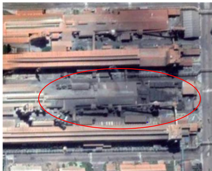
Figure 1. Bird's-eye view of an aluminum smelter.
