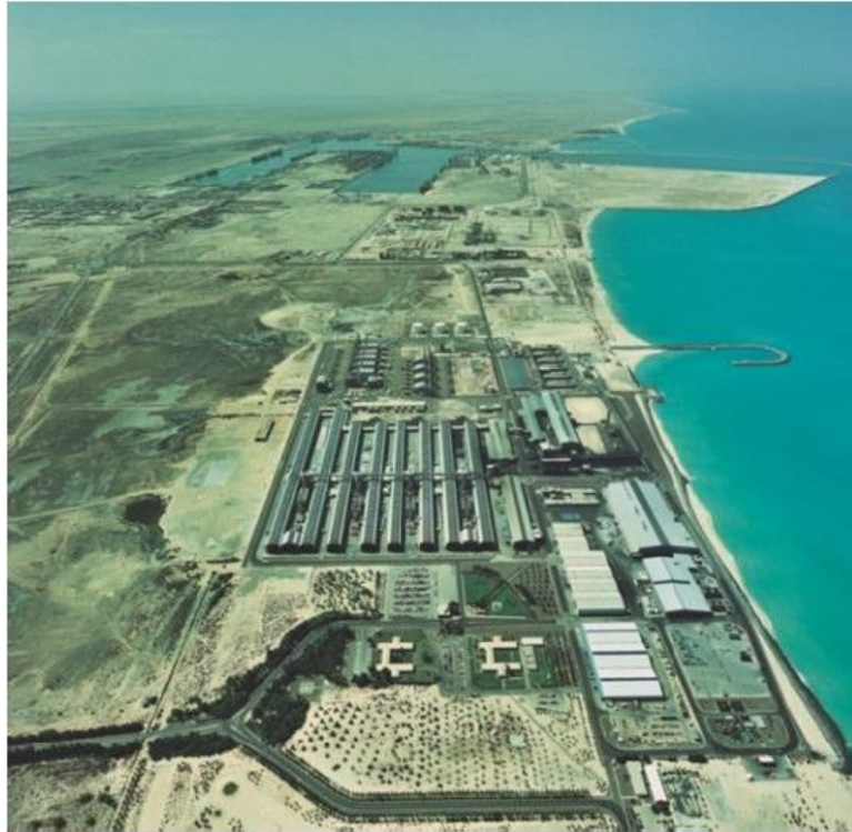
Figure 1. EGA's Jebel Ali smelter in 1990 with 4 potlines and 504 D18 cells.
