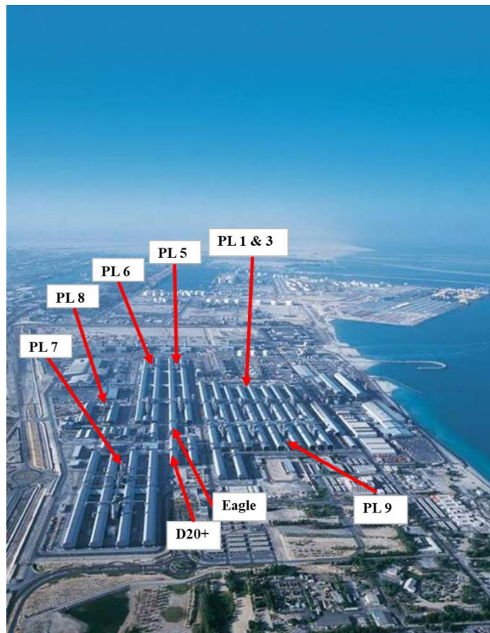
Figure 2. EGA's Jebel Ali smelter in 2022 with 7 potlines, 6 cell technologies, 1577 cells.
