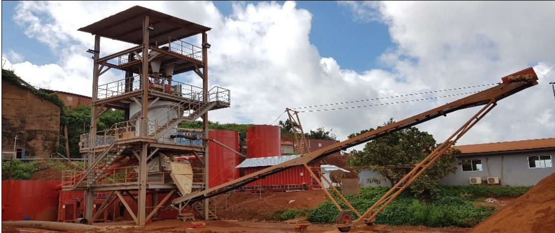
Figure 13. Processing plant fresh tailings.
