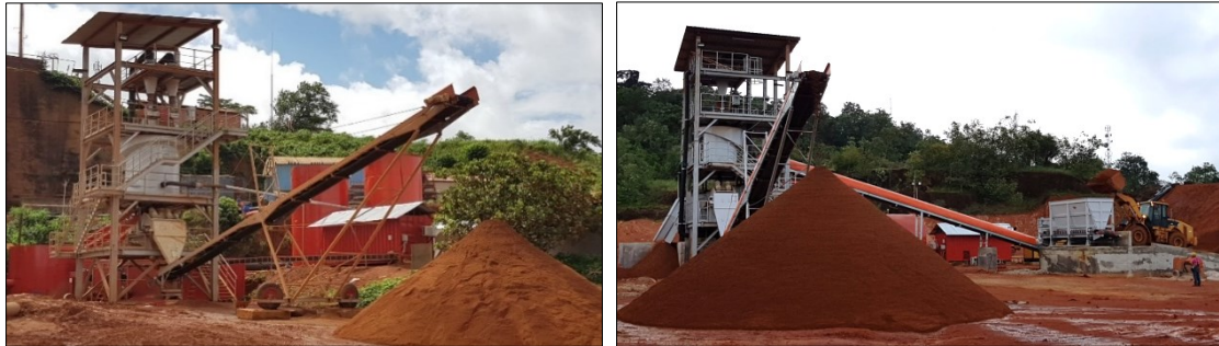
Figure 11. Processing plant fresh tailings (left). Figure 12. Processing plant stock tailings (right).
