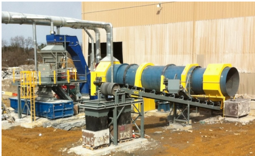
Figure 18. RT 108 System with magnetic separation.
