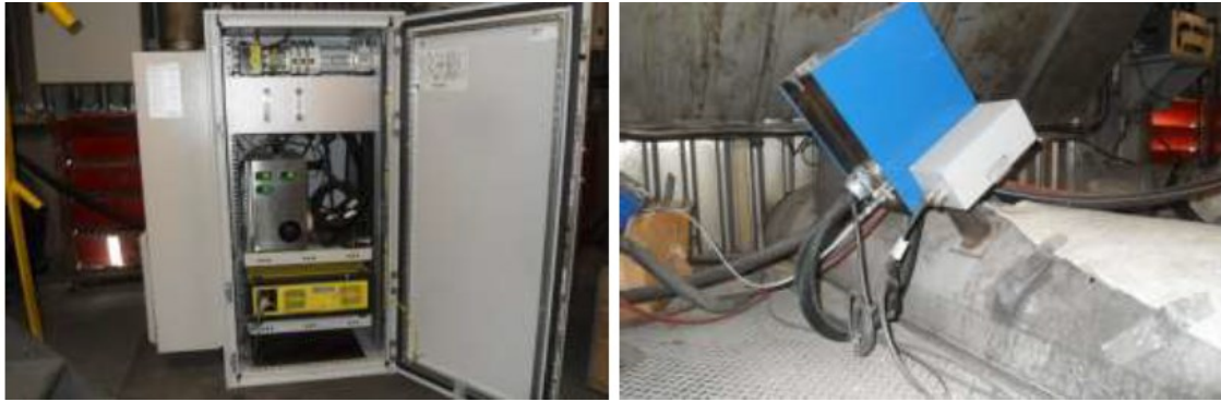
Figure 8. Online monitoring of PFC emissions. Left: electronics cabinet, Right: spectrometer.
