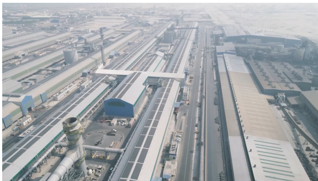
Figure 1. Aerial view of ALBA smelter with Line 6 in the center.
