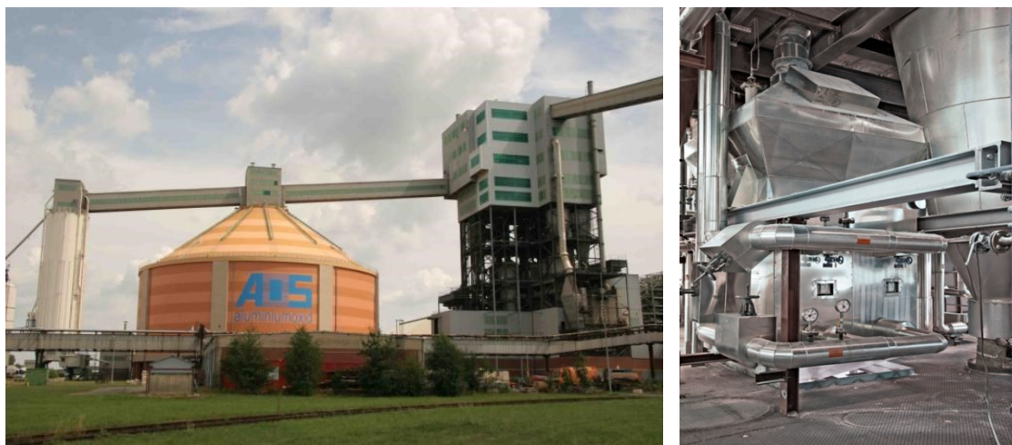
Figure 4. The calcination plant and storage silo at AOS Stade (left) and the hydrate dryer vessel installed at Calciner 2 (right).
