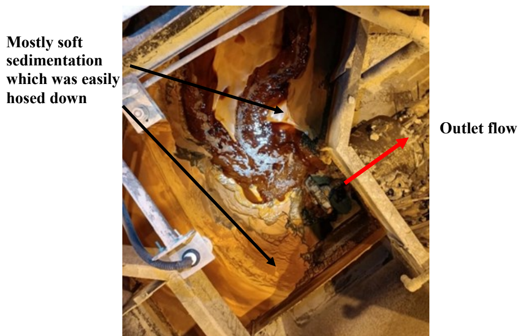
Figure 9. Photograph of scale and sediment in Y-Flume from H row, modified design.
