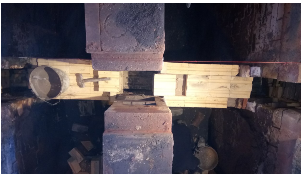
Figure 13. Headwall reconstruction around old fluewalls
