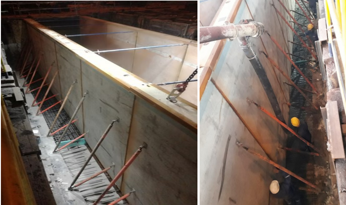
Figure 11. New prefabricated walls and pouring of new raft
