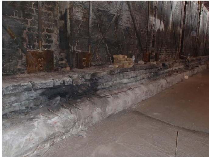
Figure 9. The existing raft condition after cleaning
