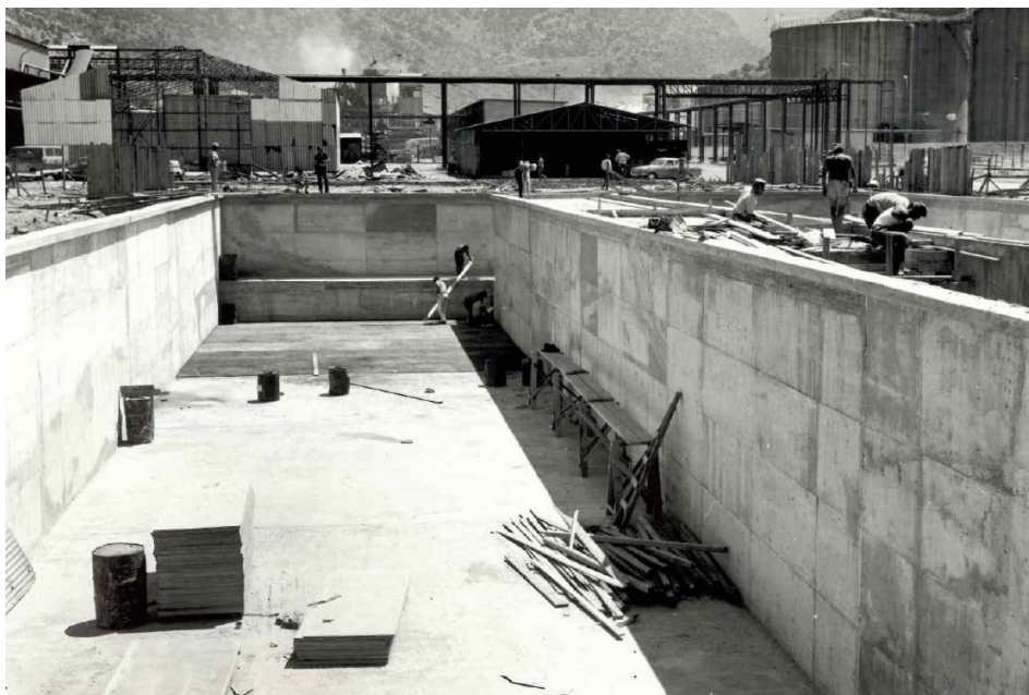
Figure 1. Aluminium of Greece concrete casing during furnace construction (1970)
