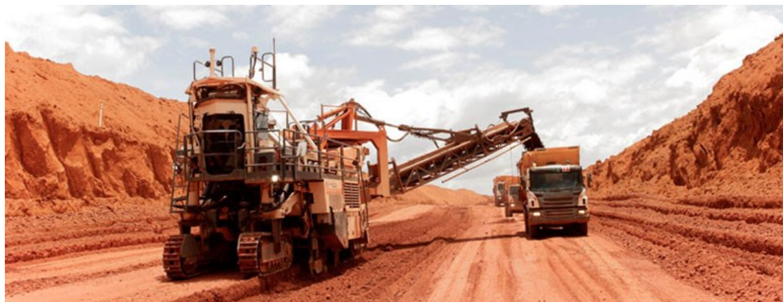
Figure 1. Surface miner loading trucks in a mining area.
