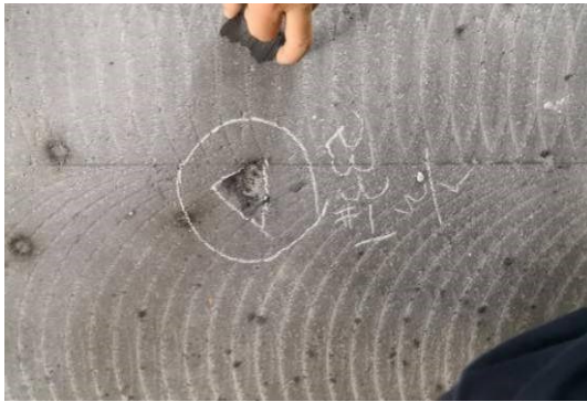
Figure 3. Cracks in Pot #1540 A16.
