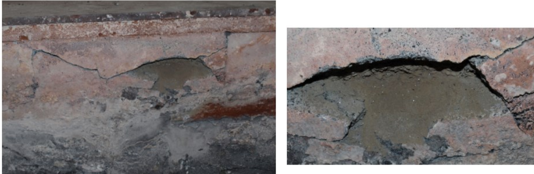
Figure 2. Example of severe degradation due to bad quality sidelining material. Plant B.
