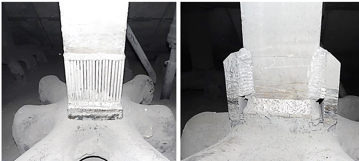
Figure 9. Technical solution to improve the connection reliability.
