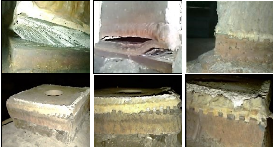
Figure 3. Examples of breakdown of the Fe-Al bimetallic joint of the RA-400 pot.
