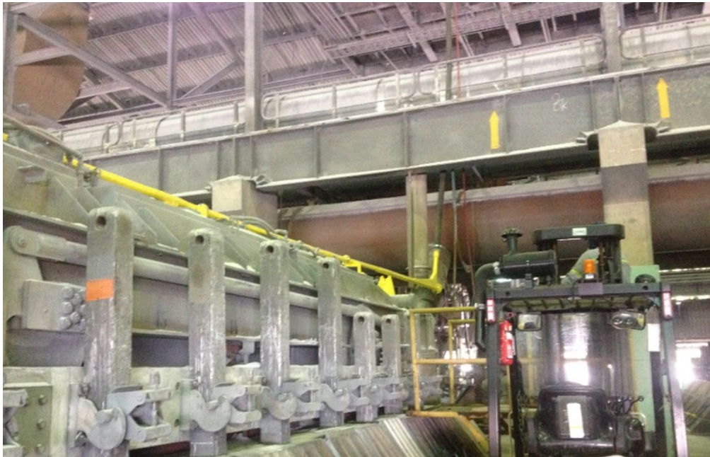
Figure 2. Multi-outlets nonmetallic fluidized pipeline – during erection time.
