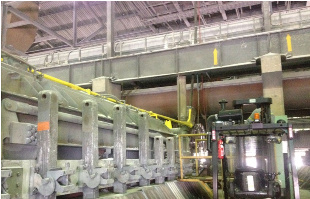
Figure 2. Multi-outlets nonmetallic fluidized pipeline – during erection time.
