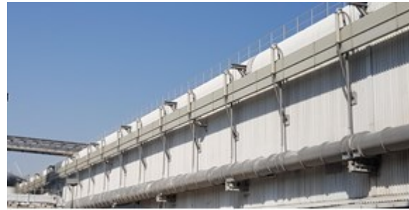
Figure 6. EGA Al Taweelah Potline 1 HDPS system.
