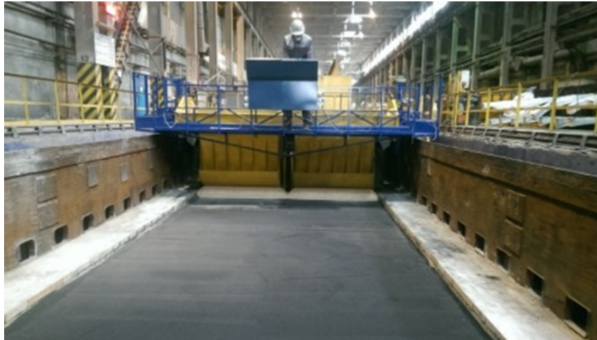
Figure 4. General arrangement of equipment for loading and laying ULM.
