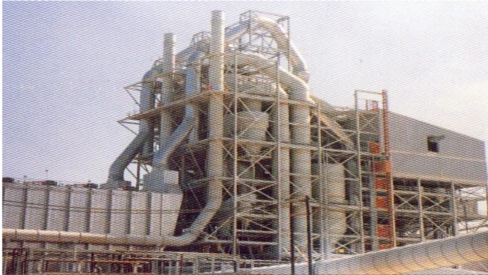
Figure 2b. Integrated GSC with reduced tower height, Sherwin alumina.
