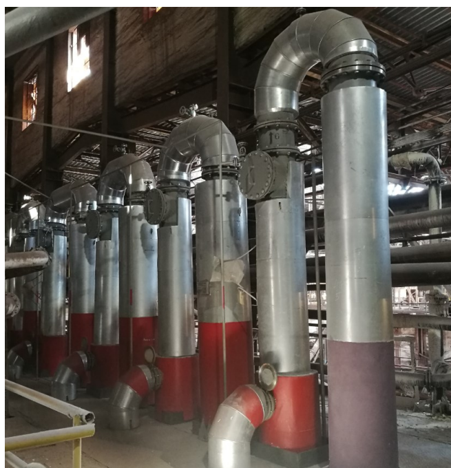
Figure 4. Assembled element shell and tube heater.
