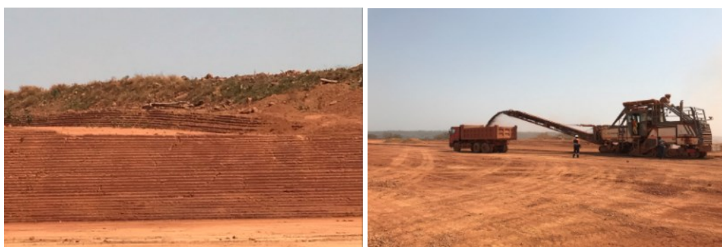
Figure 8. Mining at Dian-Dian using surface mining equipment.
