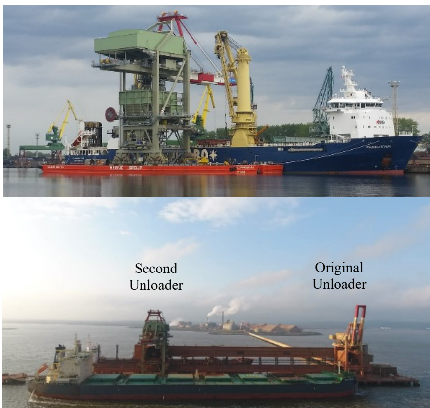
Figure 10. Second unloader before shipping and after installation completion.
