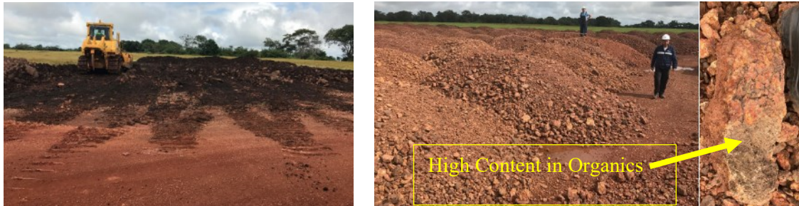
Figure 3. Stripping and Segregation of Top Soil, Overburden and high TOC bauxite.
