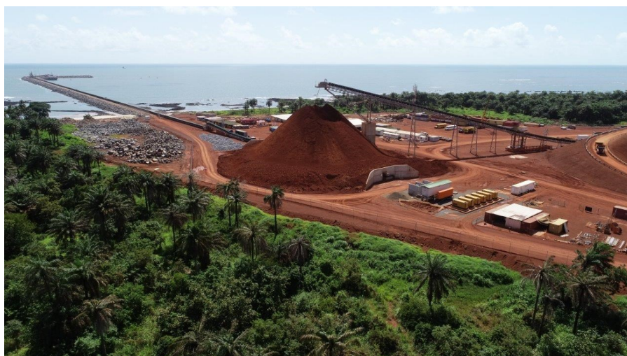
Figure 3. Stockpile and causeway facilities.
