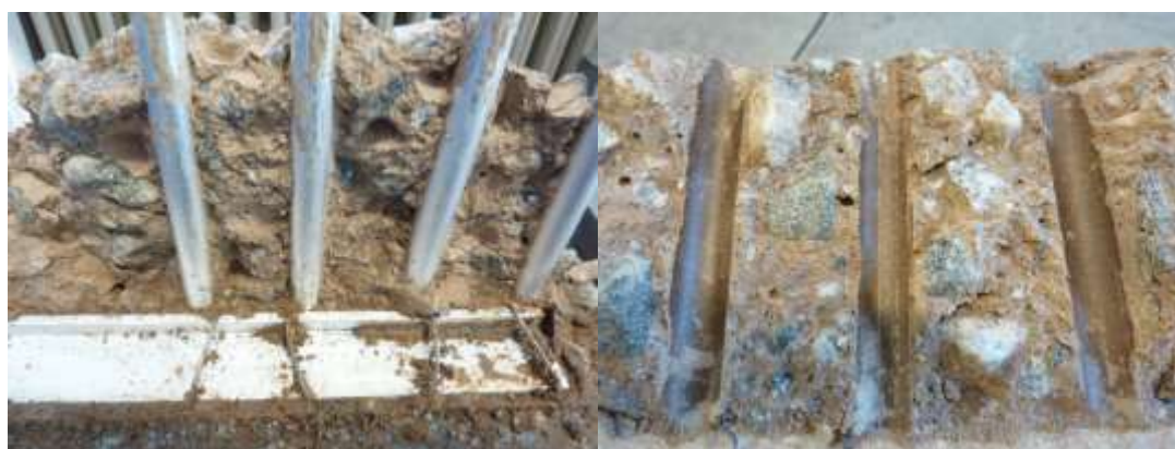
Figure 9. Aluminum reinforcements exposed (left) and their imprints (right) in concrete after 40 days in moist conditions showing no sign of corrosion.
