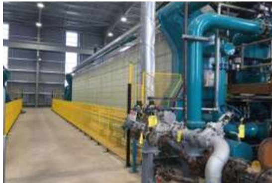
Figure 6. Plate filter press
