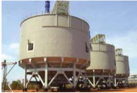
Figure 2. Paste thickeners
