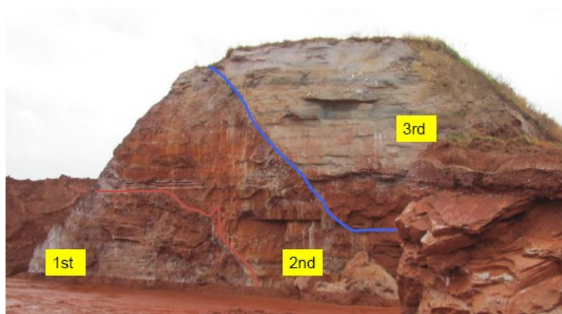
Figure 3. Stages of building of the embankment [7].
