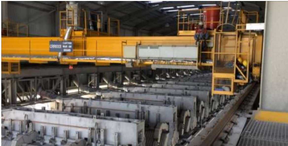
Figure 8. Rail inspection car being used in one of the section for rail inspection.
