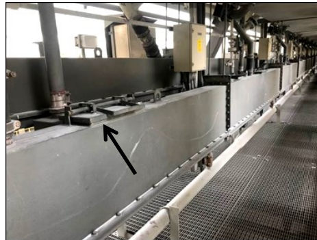
Figure 1. GTC primary alumina airslide with sampling locations.
