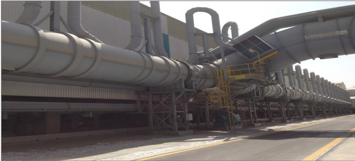
Figure 6. Hairpin type duct cooling system with air dilution damper in Ma'aden GTC.
