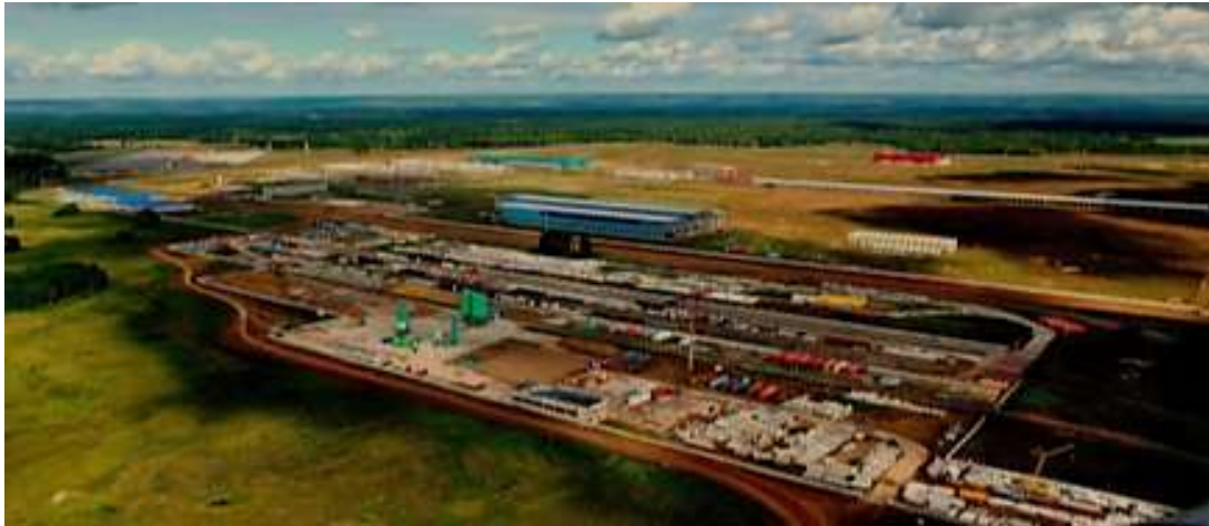
Figure 3. Taishet Aluminum Smelter (RA-400, RA-550 technologies) – in construction.
