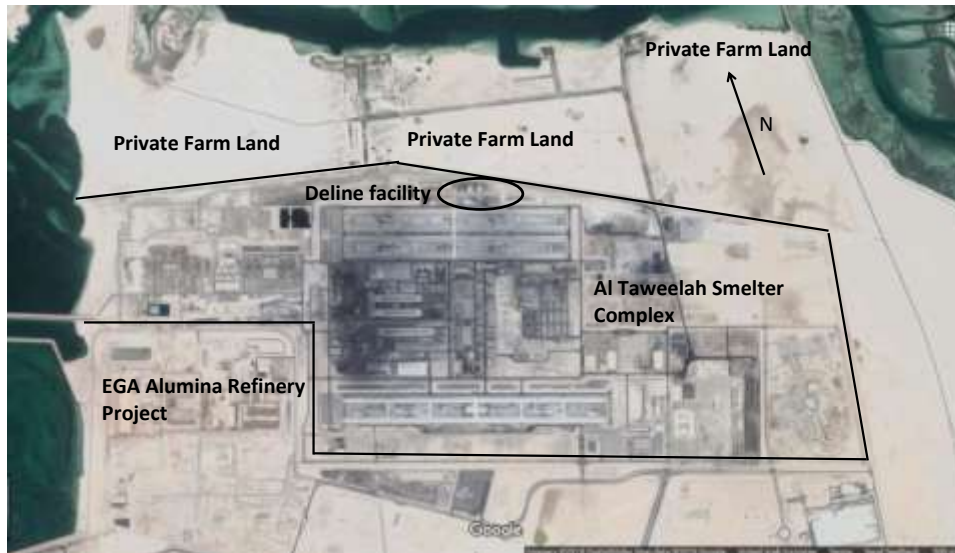
Figure 6. Al Taweelah aluminium smelter complex.
