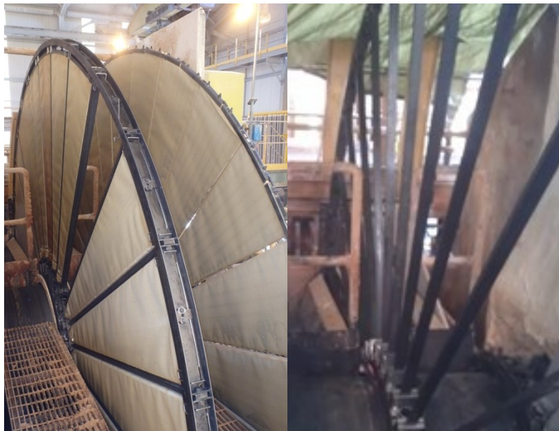
Figure 5. Spoke wheel construction
