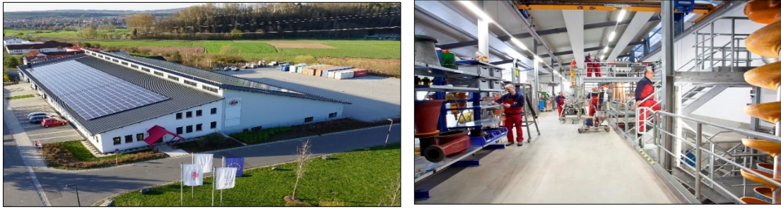
Figure 1. (a) Test center and warehouse; (b) Test center extract from the main hall.
