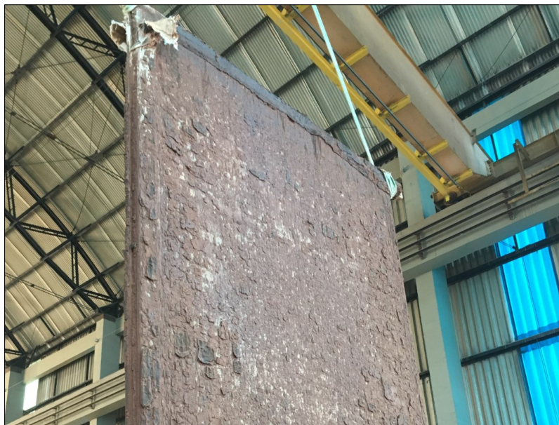
Figure 2. Scale on the filter bag during filter refurbishing.
