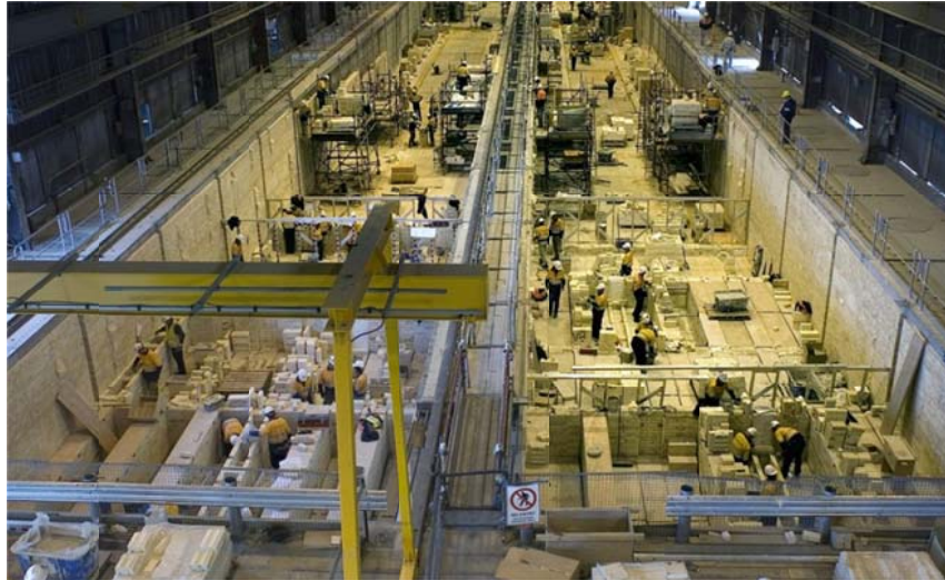
Figure 3. Workers during a complete furnace reline
