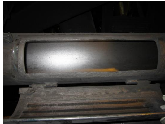
Figure 5. Ventilation duct after fine coke injection point implementation
