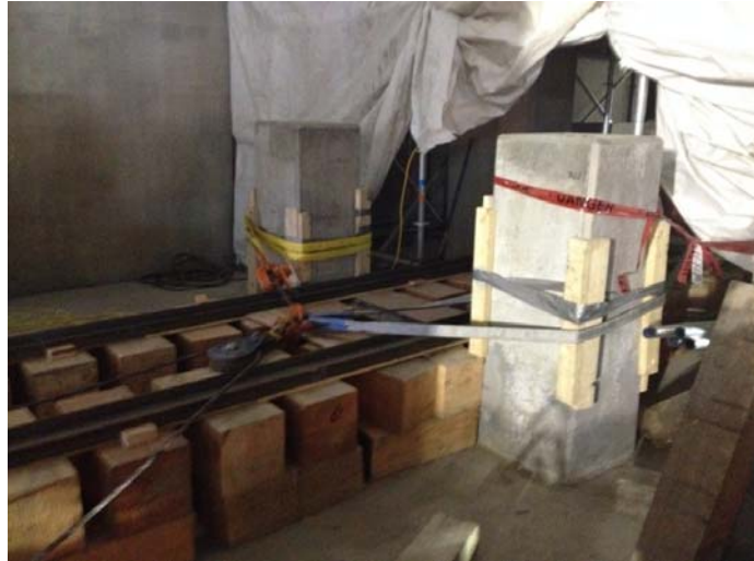
Figure 14. Rail system used to move the modules on site [2].
