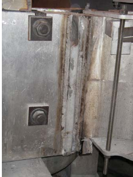
Figure 7. Complete ESW welding joint.
