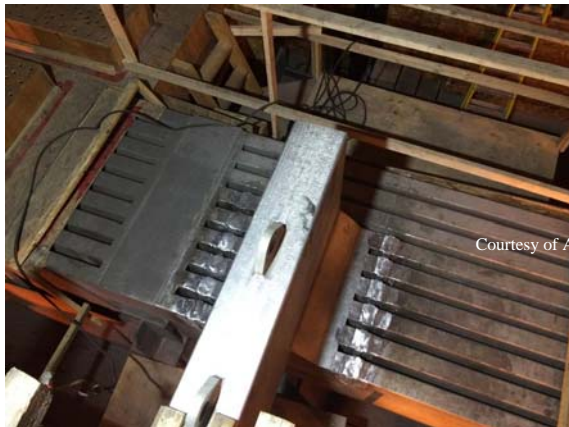
Figure 20. Preassembled modules as fabricated [3].
