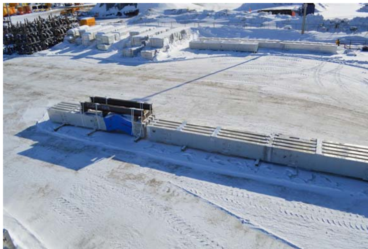
Figure 13. Modules ready for delivery to Kitimat [2].
