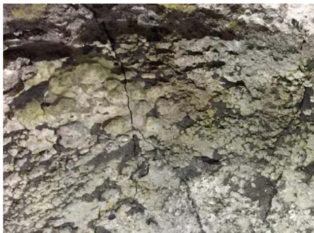
Figure 2.7. Pitting on the carbon cathode surface.
