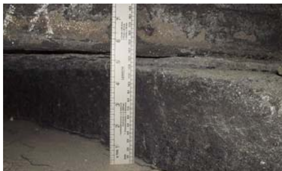
Figure 5. Condition of CDBM after 2,331 days of operation, Cathode of Cell A.
