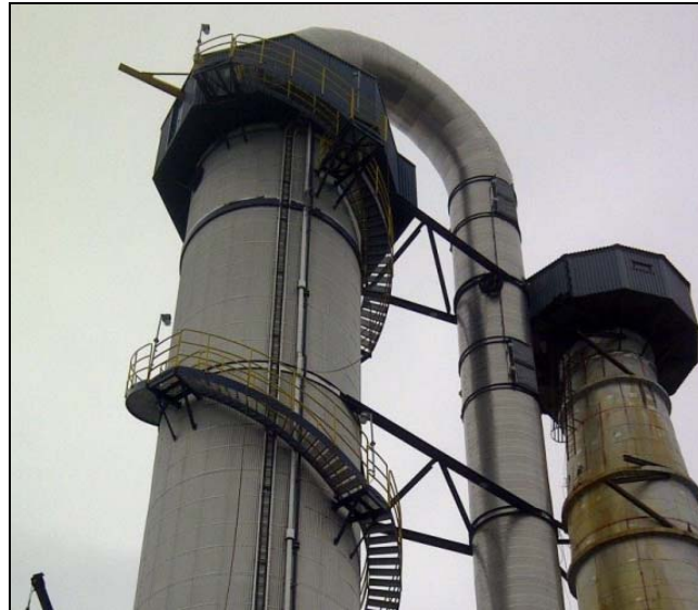
Figure 9. New conditioning tower alongside existing tower.
