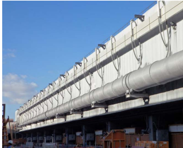
Figure 11. Basic of Alfeed. The distribution air slide hangs on the pot room wall and feed pot airslides.
