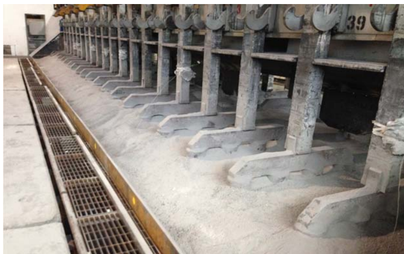
Figure 8. Prepared cell ready for preheating.
