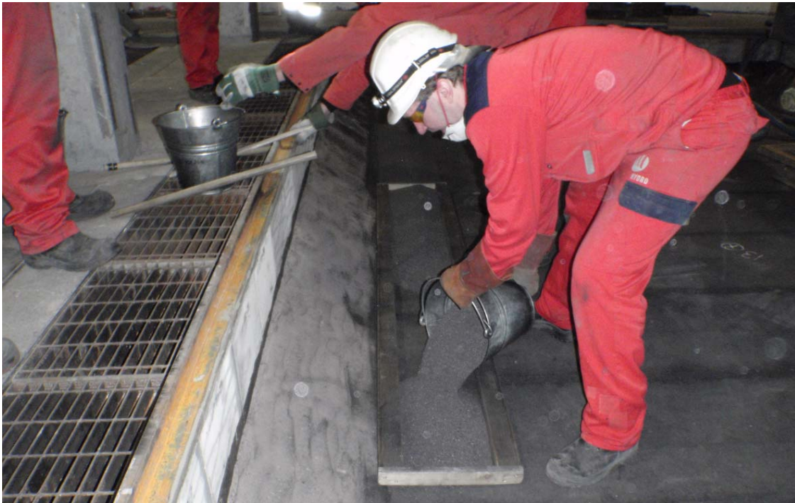
Figure 5. Laying graphite stripes close to the side of the cathode.
