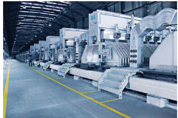
Figure 2. D18+ Technology test cells in Potline 1.
