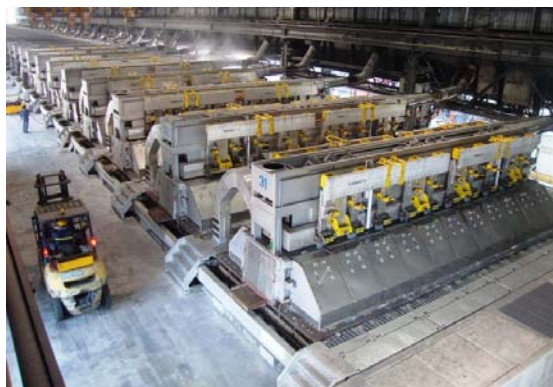
Figure 13. Section 2 under preheat.
