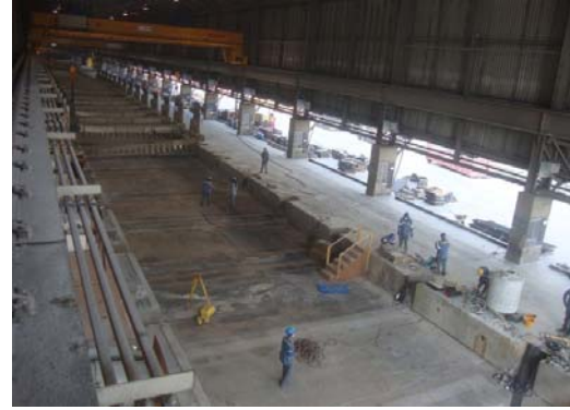
Figure 8. Potroom after D18 busbar removal.
