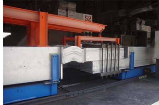
Figure 5. Bypass busbar in situ.
