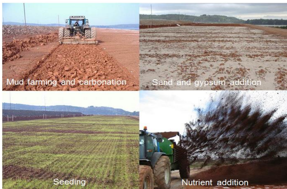
Figure 9. Steps in the rehabilitation and revegetation of deposited red mud
