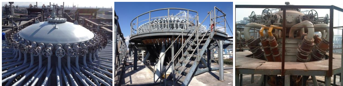
Figure 11. Examples of the basic design of distributors for alumina refineries
