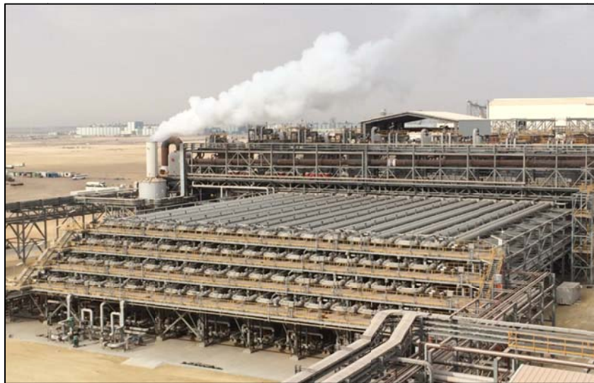
Figure 5: Ma'aden Hybrid Tube Digestion Facility
