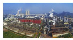
Aluminium Smelter - Guangxi Hualei New Material Co., Ltd. Founded in 2015, Guangxi Hualei New Material Co., Ltd. is an integrated enterprise specializing in primary aluminum production, power generation, and aluminum processing. With an annual capacity of 400,000 tons of primary aluminum, it leverages cutting-edge 500KA cell technology,
