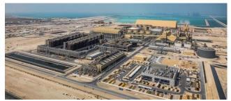
Al Taweelah smelter has a capacity of 1.5 million tonnes per year, from 1266 reduction cells using EGA technology. Potline 3 is the longest potline in the world.
